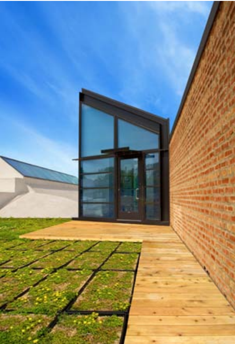
GREEN ROOF TERRACE AT KINOWERKS, CHICAGO, IL
