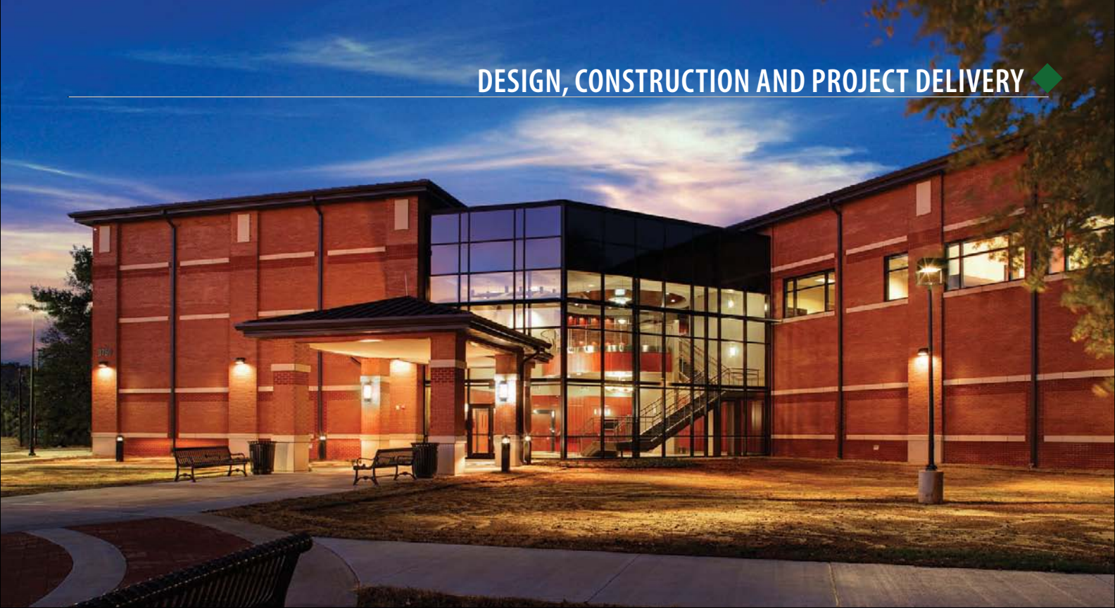
The exterior of the 81,500-ft 2 NCTER mixes classic brick veneer and metal roofing to merge the facility with adjacent structures, while the interior main entry includes a spacious, two-story lobby and grand stairway that conveys a sense of procession and dignity. PHOTO BY PETER MALINOWSKI, COURTESY OF VOA ASSOC. INC.
